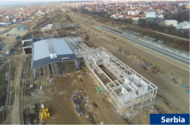
Serbia Project Services Client Construction of the new technical and passenger railway station, Zemun Construction; Procurement; Srbija voz
