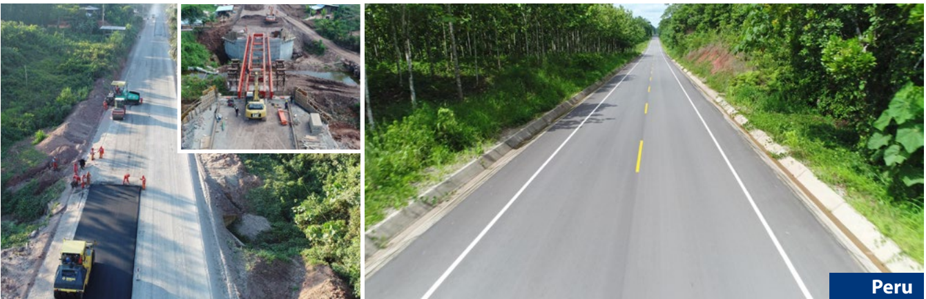
Peru ProjectRehabilitation and reconstruction of a road section Puerto Bermudes - Ciudad Constitucion ServicesUpgrading, expansion and asphalt paving of the road section and rehabilitation of the existing and construction of three new bridges ClientProvias Nacional del Ministerio de Transporte y Comunicaciones
