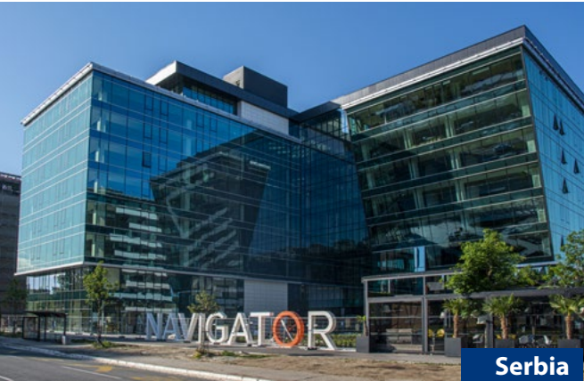
Serbia Project Services Client Administrative building “Navigator Business Center 2” Works execution; GP SEVEN d.o.o. Beograd for MPC Properties, Belgrade
