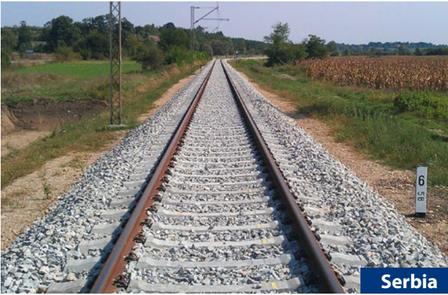
Serbia Project Services Client Railway section "Straževica tunnel (enter) - Jajinci - Mala Krsna", on (Belgrade) Rakovica - Railway Hub K1 - Jajinci - Mala Krsna - Velika Plana railway and railway station "Mala Krsna" Execution of construction and electric works; Infrastrukture železnice Srbije, Beograd
