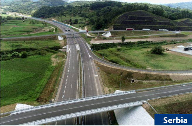
Serbia Project Services Client Highway E763, Section V: Lajkovac-Ljig and Brančiči tunnel Construction works Serbian Ministry of Construction / China Shandong International Economic & Technical Cooperation
