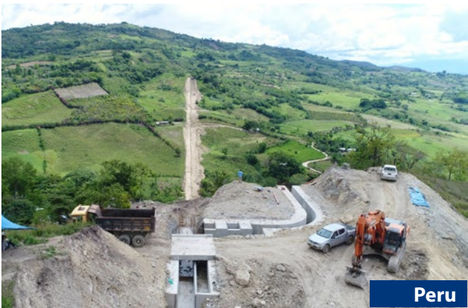
Project Services Client Irrigation system in San Antonio, Huarango, Haen Works execution Ministerio de Agricultura y Riego (MINAGRI), Peru
