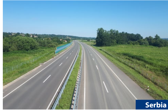
Serbia Project Services Client Highway E763, Section IV, Ub - Lajkovac Works execution; China Shandong International Economic & Technical Cooperation
