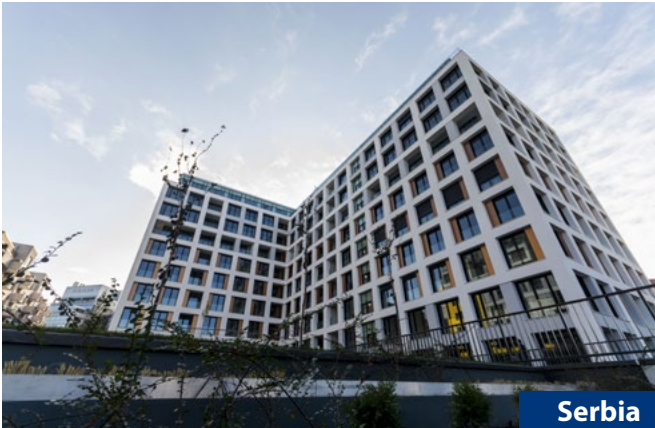
Serbia Project Services Client Residential and commercial building Park 11, Block 11a, New Belgrade Urban Project; Design; Construction; Energoprojekt Park 11 doo Beograd
