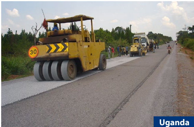
Uganda ProjectReconstruction of Mityana - Mubende road 86km and upgrading of town roads ServicesWorks execution ClientUganda National Roads Authority (UNRA)
