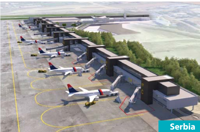
Serbia Project Services Client Nikola Tesla Airport, Belgrade - Refurbishment and extension of the terminal building with ancillary facilities Design - the entire design documentation (all stages); VINCI AIRPORTS SERBIA
