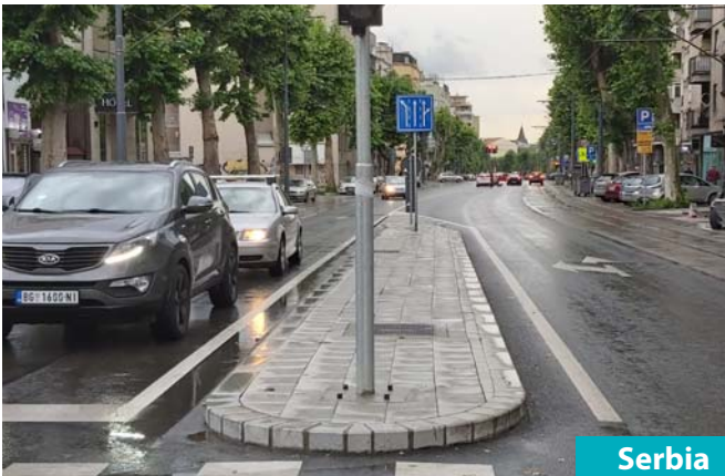
Serbia Project Reconstruction of the Belgrade streets (kraljice Marije, 27. Marta, Džordža Vašingtona, Cara Dušana) Services Works execution; Client City of Belgrade, Secretariat for Investment
