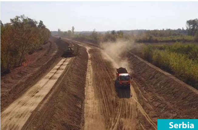
Serbia Project Reconstruction of Flood Protection System – Mačva Services Construction supervision; Client Delegation of the European Union to the Republic of Serbia
