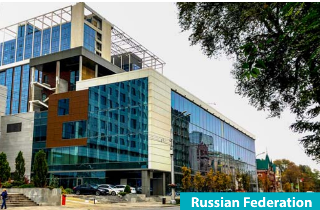
Russian Federation Project Services Client Internacional conference center and hotel “Hyatt Regency Rostov Don-Plaza” , Phase II, Rostov on Don General contractor - structural, MEP & finishing works; OOO MKC-RosEvroDevelopment
