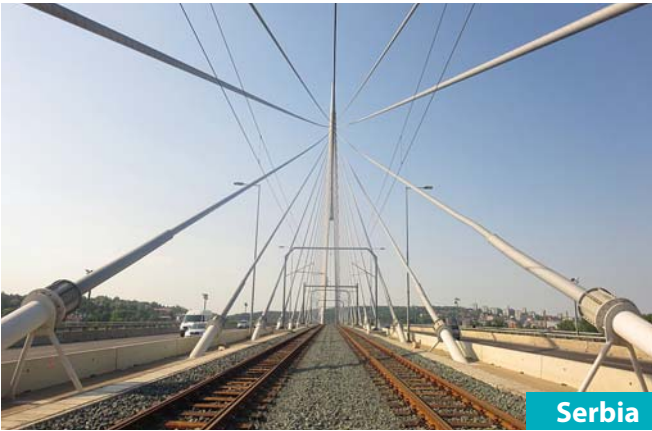
Serbia Project Construction of the tram-railway over the Ada bridge in Belgrade Services Works execution; Client Belgrade City Government
