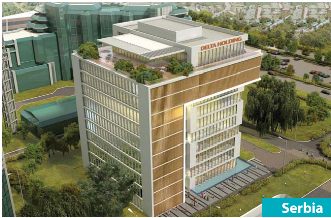
Serbia Project Services Client Construction of the administrativ building Delta Headquarters, Belgrade General contractor - execution of structural, MEP & finishing works NBGP Properties d.o.o.
