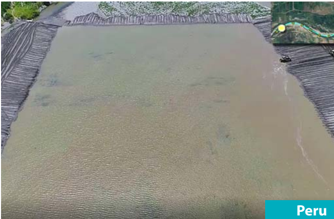
Peru Project Preventive cleaning of the river-bed of Chira river Services Formation of "Pilot" channels along riverbed 100 - 150 in width on 2 sections ( from km25 to km 40 and from km 52+900 to km 53+670); Client MINAGRI Ministerio de Agricultura y Riego
